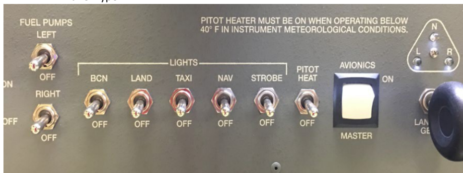
Image 40: Center of Lower Switch Panel Type 1, 2, & 3
